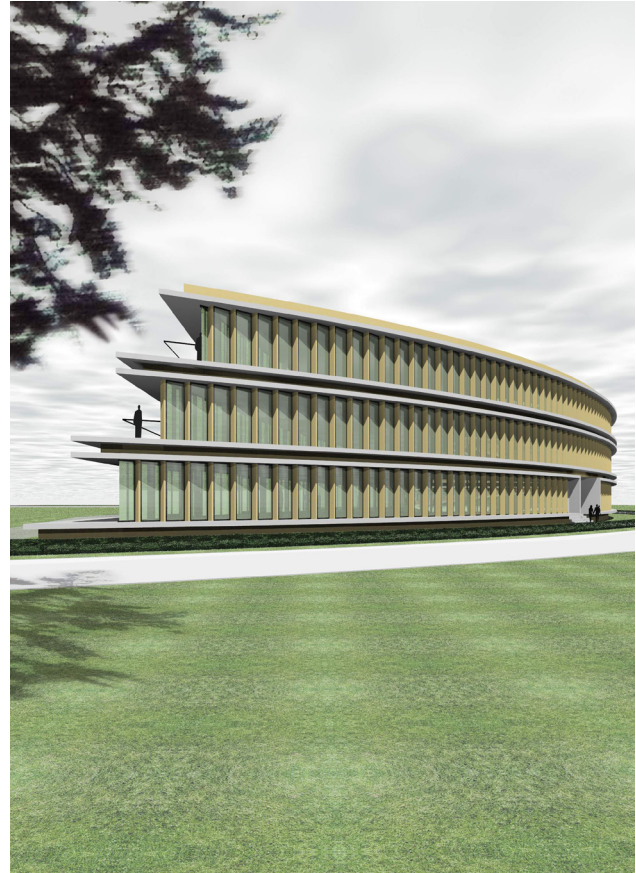
South-east view: The curved facade is constructed with simple flat floor to ceiling glass windows in a sawtooth pattern. For natural ventilation the reveals can be opened instead of the windows.
